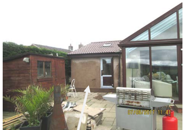
the extension looking from the rear
