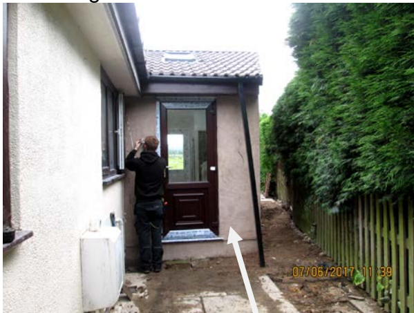
the side utility extension from the front
